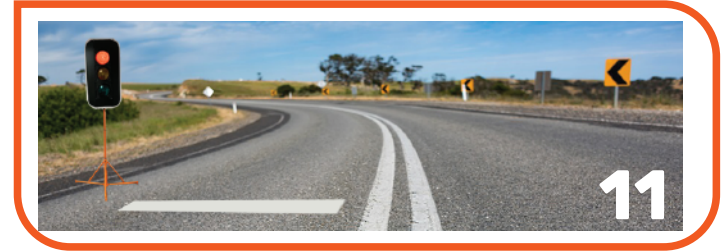
ADJUST ANGLE OF TRIPOD WITH ADJUSTMENT LEG - APPLY BALLAST / SANDBAGS TO STABILISE
